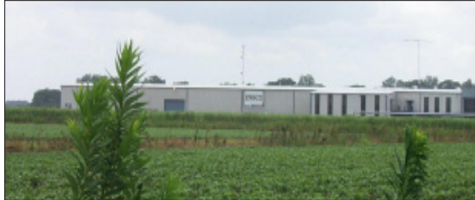
Light industrial warehousing is being developed outside of the urban fringe. This is beginning to cause conflicts with rural residences in the area.
